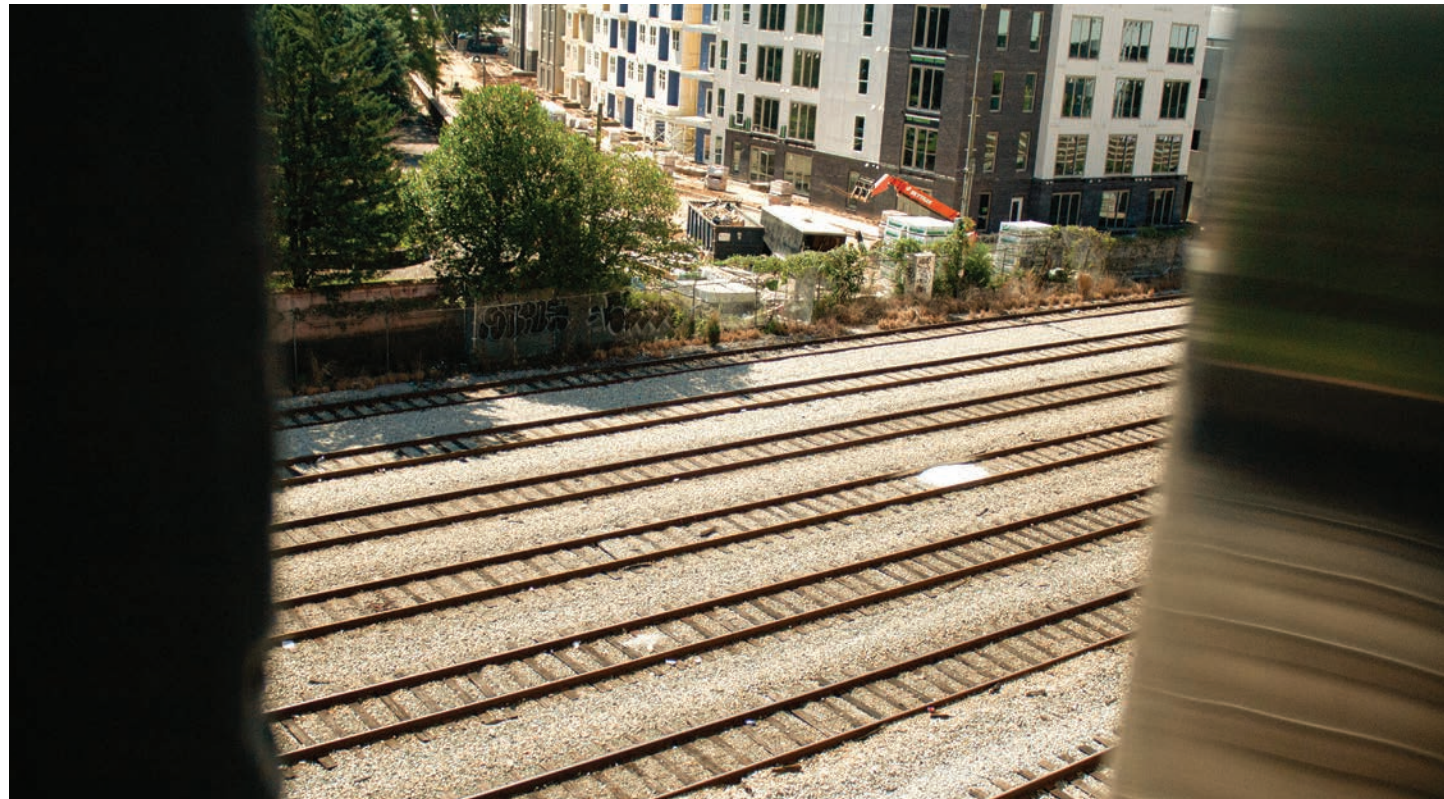
View of adjacent rail at the MLK Jr. MARTA Station // Photo by MEGAN MINNEAR
